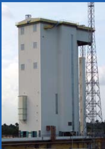
Vega's mobile launch gantry approaches the umbilical mast during its rollout test at the Spaceport
