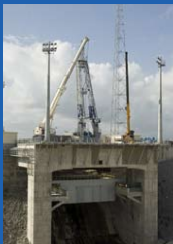
An umbilical mast is installed on Soyuz' new launch pad at the Spaceport in French Guiana
